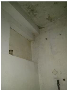
Detail strop v kuchyni
